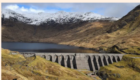
Cruachan hydro electric power station © Jeff J Mitchell/Getty Images
